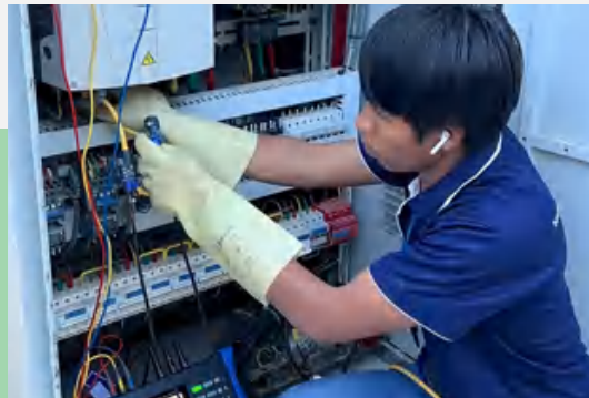
TeraHop Thailand Exhaust Fan Speed Adjustment
